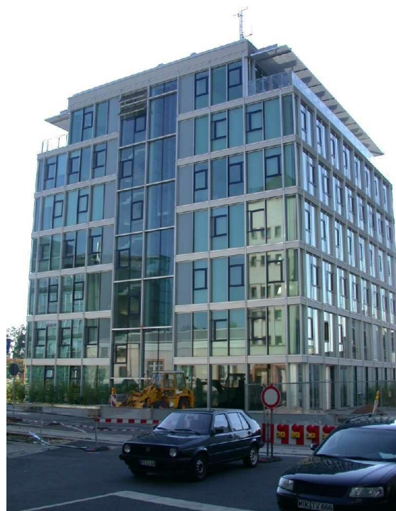
Figure 1: Low energy office building of the port utility of Frankfurt a.M. (Heating energy consumption = 35 kWh/m 2 a)
