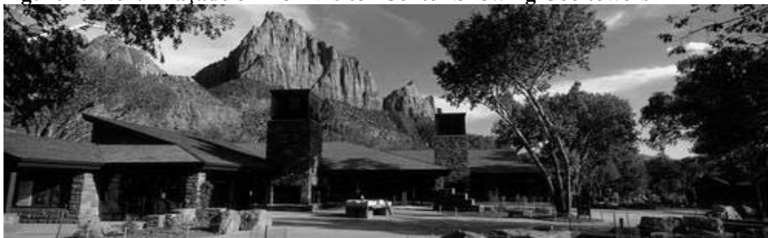
Figure 2. North Façade of Zion Visitor Center Showing Cooltowers
