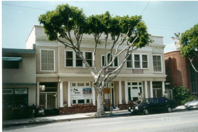
Figure 1. Photograph of Site with Existing Building
