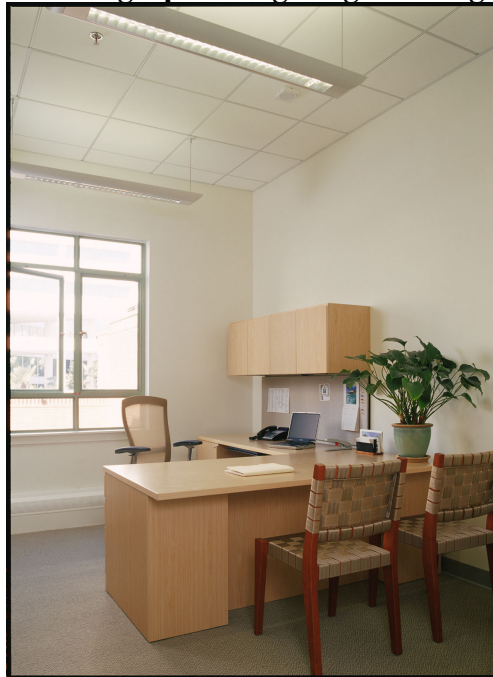
Figure 5. Photograph of Lighting Building System 4
