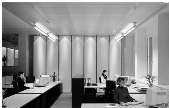
Figures 2-4: The progression of lighting via the indirect component, the individual adjustment of specific lighting situations such as the direct lighting for the workplace and the surprising effects of the strip light on the wall motivate employees in the office; the sequence of lighting changes is recorded in a story board.
