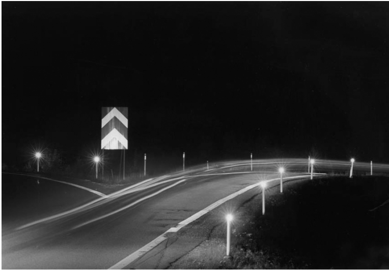
Figure 1. The road junction at night. Each pole has an active LED unit, as well as a reflective background coating.
