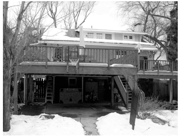
Figure 3. The front of this home faces west toward Boulder's mountains, the back, east. Note patterns of snow melting, suggesting voids in attic insulation.
