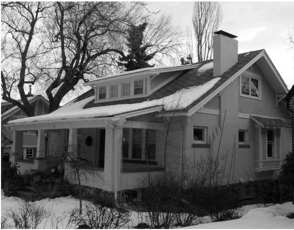
Figure 3. The front of this home faces west toward Boulder's mountains, the back, east. Note patterns of snow melting, suggesting voids in attic insulation.
