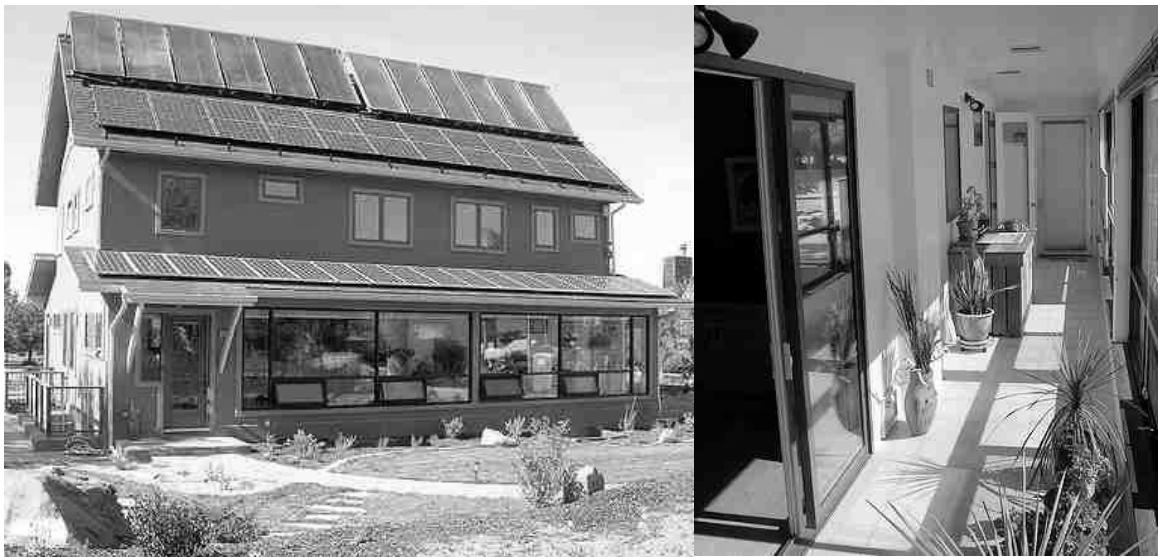
Figure 6. South elevation and solar space in “Solar Harvest” home in Boulder
