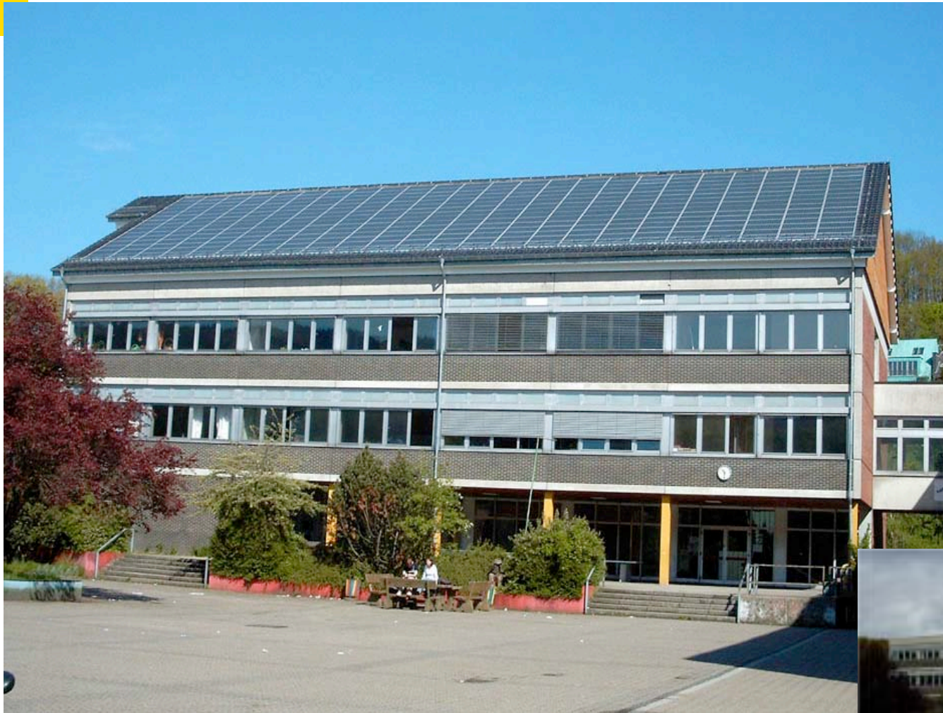
Aggertal-Gymnasium before renovation
