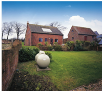
Figure 5-5. Above ground LPG storage tank 65
