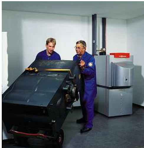
Figure 6-4. Removal of old oil boiler, new boiler in background [www.renovieren-mit- energie.de/index.php?id=26]
