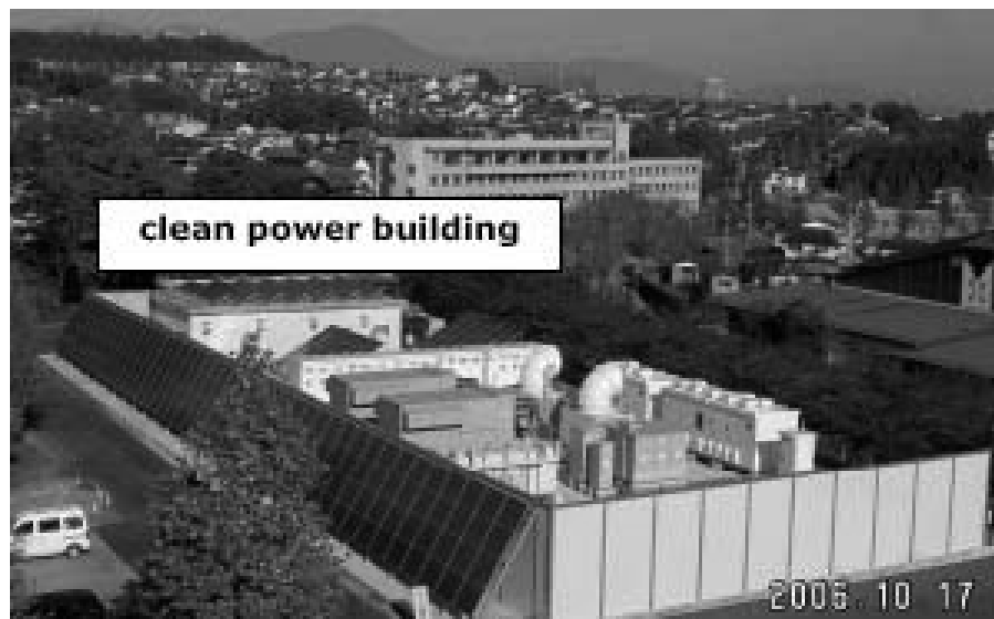
Figure 9. The Sendai Multiple SQR Microgrid Demonstration
