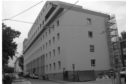
Figure 1: Pictures of the building after renovation (above) and during renovation (below).
