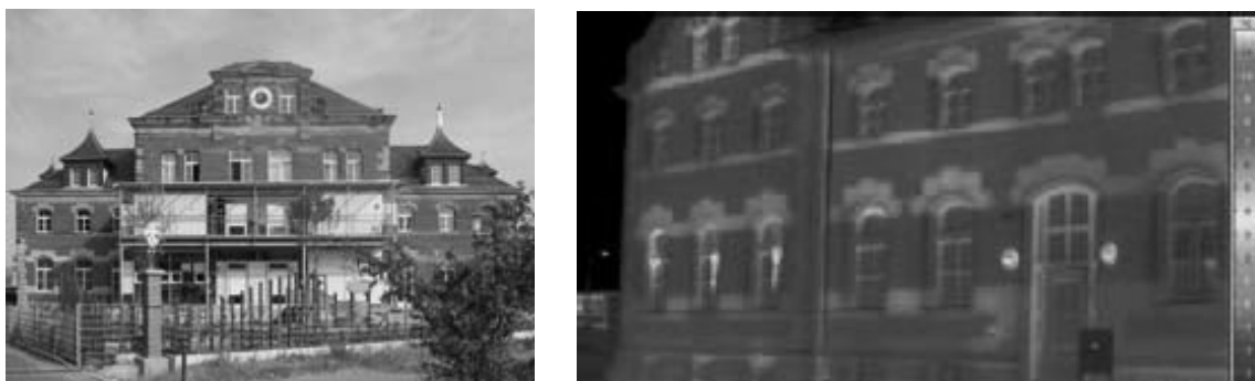
Figure 3. The refurbished building in Nuremberg, One photograph taken in the daylight and one as a result from the thermographic analysis.
