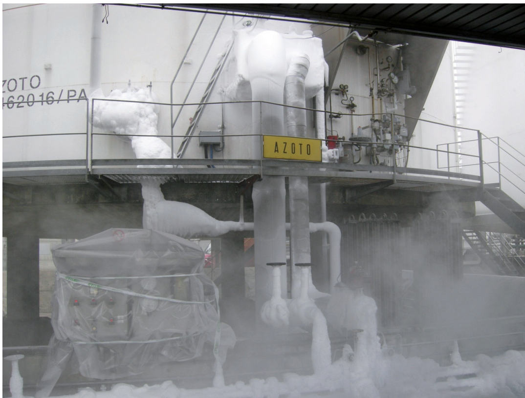
Figure 7: The control panel needed to be protected with plastic sheeting from the dripping condensation water. Extensive ice building on pipes and valves.
