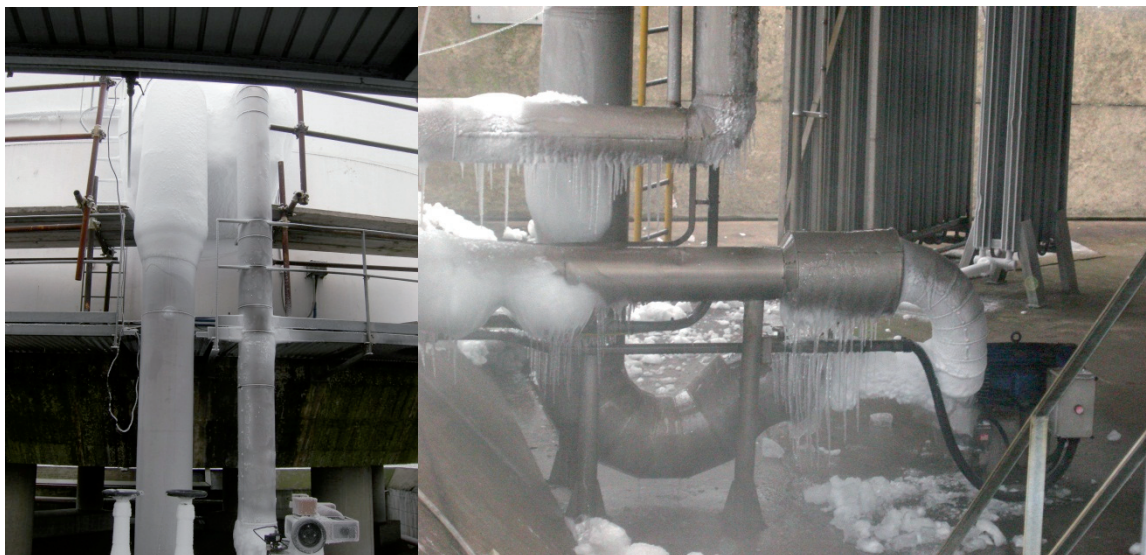
Figure 8: Broken vapour barriers and insufficient insulation caused ice to form around these pipes causing both process control problems and structural problems.
