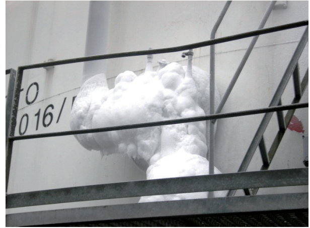
Figure 6: Valves can no longer be operated.
