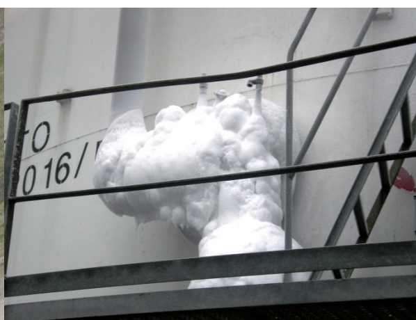
Figure 6. Valves can no longer be operated.
