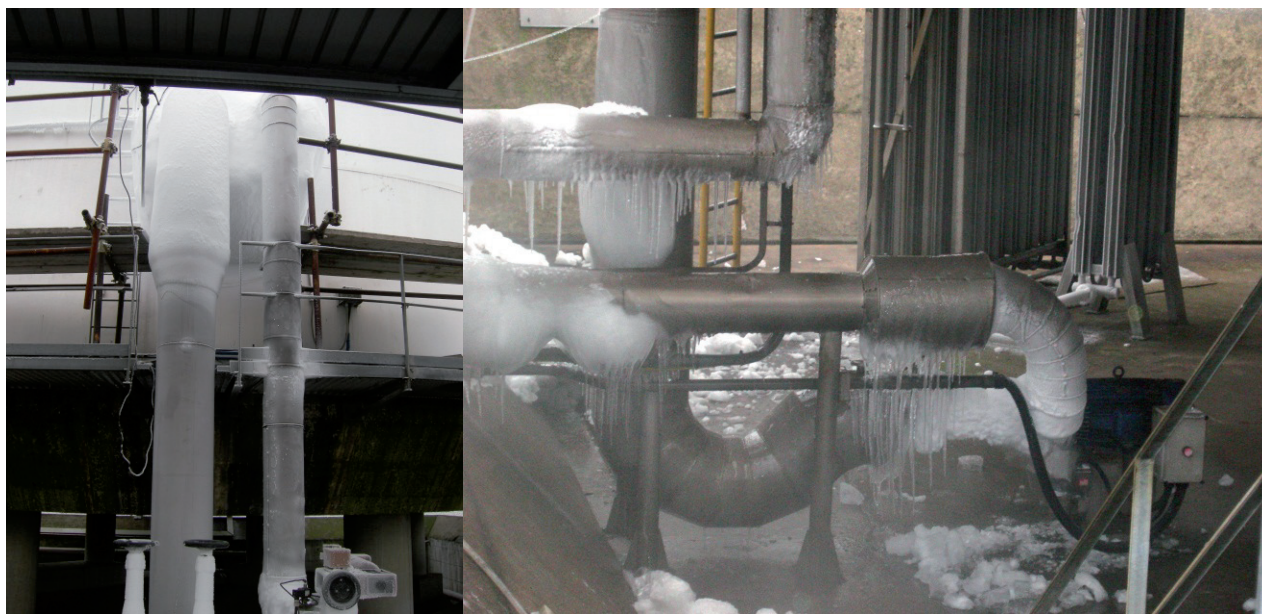
Figure 8. Broken vapour barriers and insufficient insulation caused ice to form around these pipes, causing both process control problems and structural problems.
