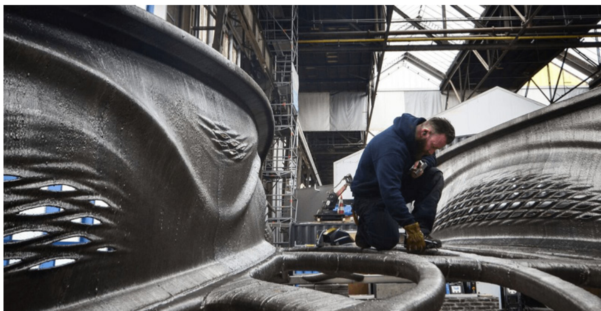
Figure 2. Quality control on the MX3D stainless steel pedestrian bridge depicting features of the design as well as patterns of welding layers reminding of structures shown in some science fiction movies (source: MX3D).
