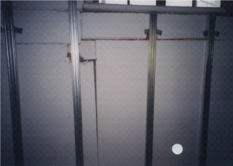
Figure 4. Internal wall insulation (expanded polystyrene) before plasterboard is fitted, showing metal fixing rails and gaps in the insulation due to poor workmanship.
