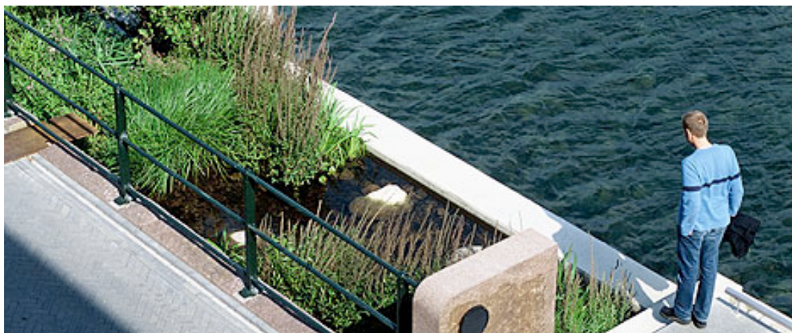
Figure 1. The Western Harbour: Detail of the open storm water system. Photo: City of Malmö.
