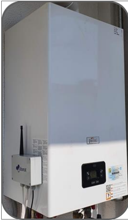
Boiler attached with the heating controller
