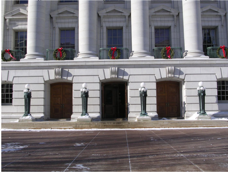
Figure 3. Outdoor Light Standards at the Capitol
