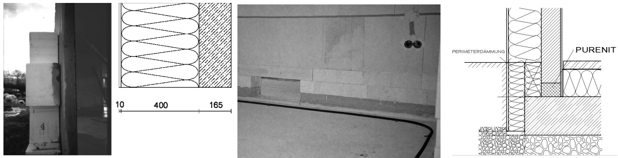
Figure 1. Left : Wall insulation at the gable wall in the CEPHEUS sub-project 01-Hannover. Right: Thermal bridge reduction at the base point in O2-Kassel.
