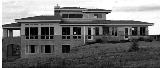
Figure 4. Tierra Concrete Home near Colorado Springs, CO, south elevation.
