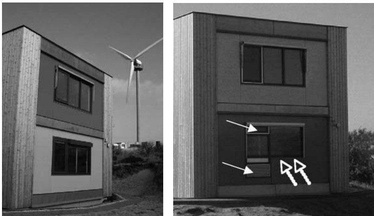
Figure 1. The four façades built, integrated in a research facility. To the left: yellow (bottom) and red façade (top). To the right: blue (bottom) and grey façade (top). The solid arrows indicate the position of the panels in the blue façade (behind grids) that can be opened for night cooling. The dotted arrows show the location of the ventilation openings, concealed under the window threshold.
