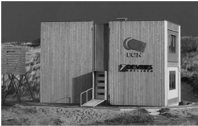
Figure 5. Research facility containing four separate rooms each holding a different façade.
