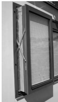
Figure 3. Detail of the yellow façade with the parallel window partly opened.
