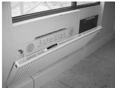
Figure 2. The Climarad ® heat recovery unit, integrated in the blue façade in combination with a radiator that can be tilted to a side for good access.
