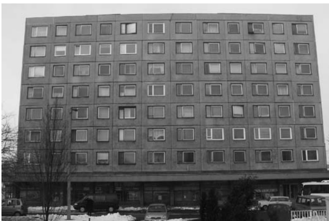
Figure 1. Southern view of the SOLANOVA building.
