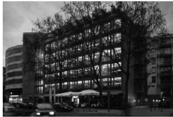
Figure 5. The building of the Helvetia insurance company in Frankfurt
