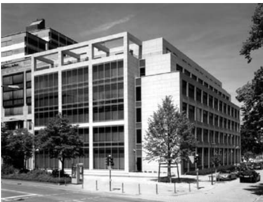
Figure 6. Outer view of Ostarkade KfW- Frankfurt am Main
