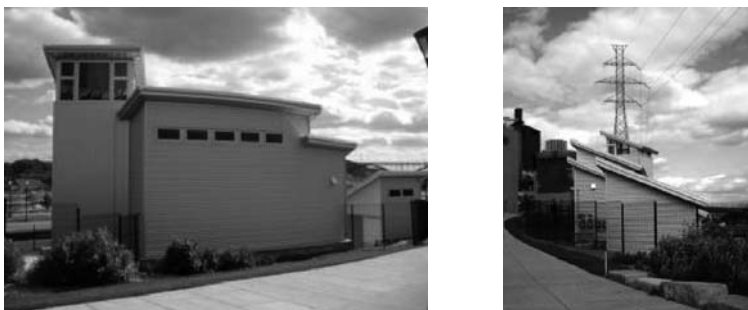
Figure 8. Science House north and west elevations showing balance of daylighting and envelope considerations.
