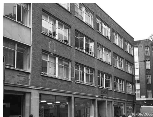
Figure 5. An office building with a high percentage of open windows.
