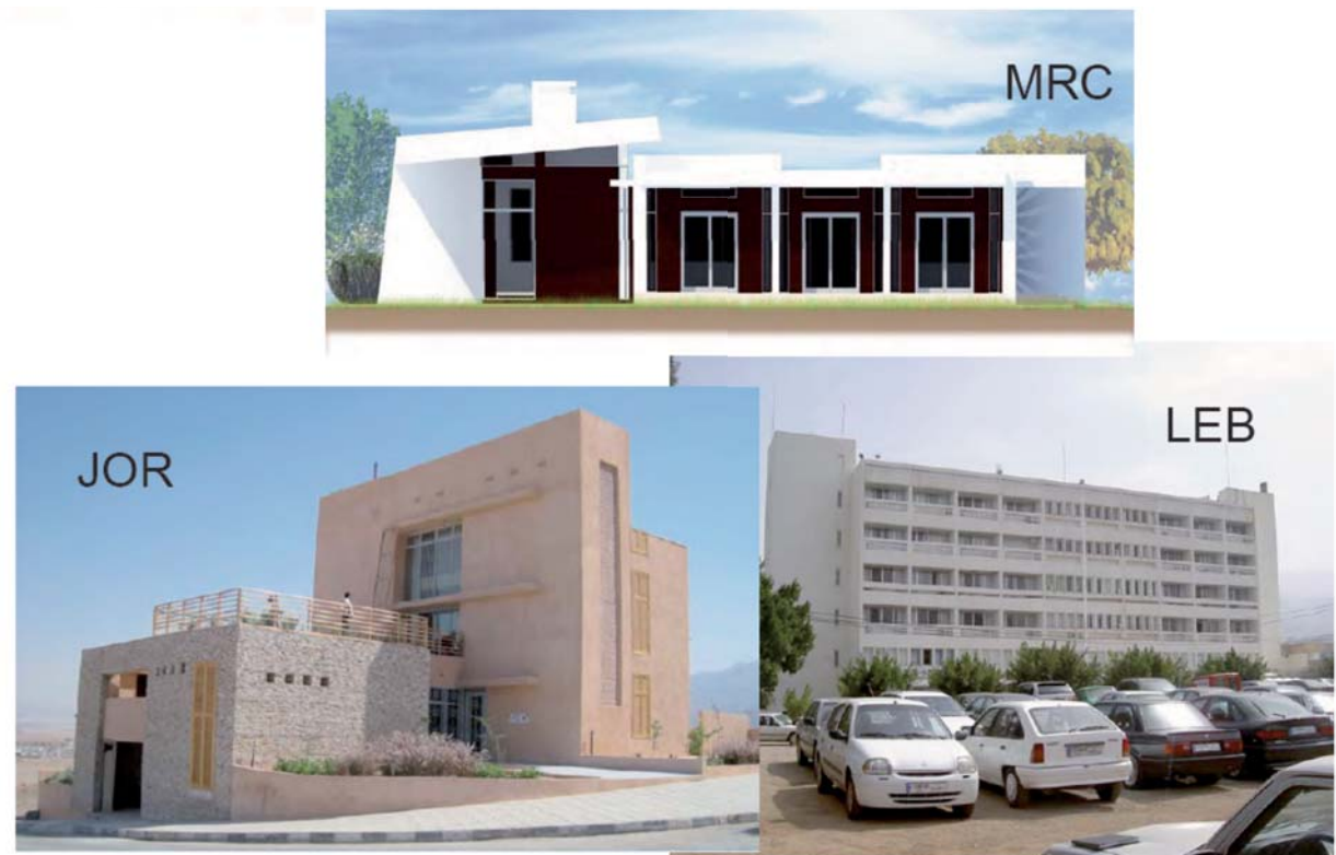
Figure 3: Pictures from MED-ENEC Pilot Projects in Morocco, Jordan and Lebanon
