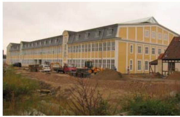
Figure 7. Ovnhallen – being retrofitted.
