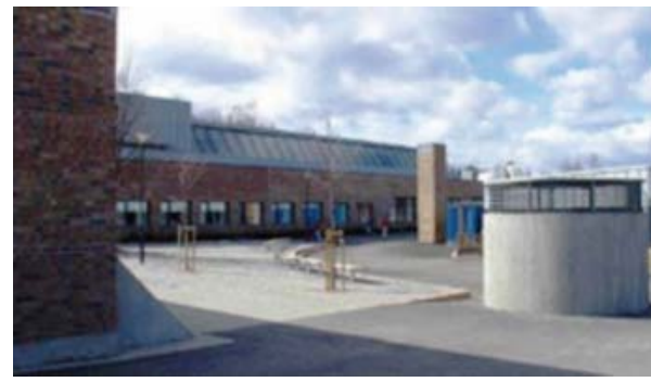
Figure 11. Pictures showing the main building before and after retrofit. The most visible features are the new daylight openings on the roof and new façades. The air inlet tower and a heat recovery unit (roof top) can be seen in the picture to the right. Architects for retrofitting: Hus Arkitekter AS. Photo left: B. Matusiak. Photo right: J. Rolland.
