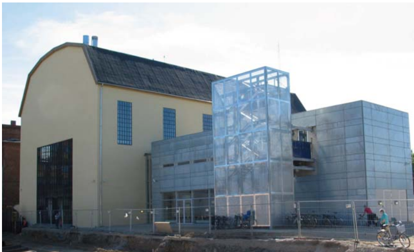
Figure 4. The building site. Ovnhallen (to the left) and Proevhallen.
