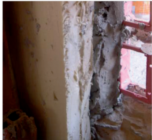
Figure 2. On site inspection in Carugate. Thick insulation layers may be seen in the surrounding walls in new constructions.
