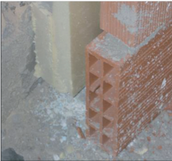
Figure 2. On site inspection in Carugate. Thick insulation layers may be seen in the surrounding walls in new constructions.
